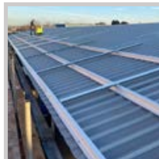
Over Roofing & Cladding
